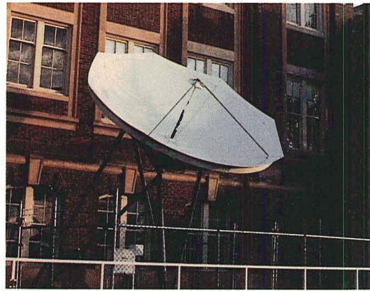
Relatively inexpensive satellite reception dishes, like this one at a Stillwater (Oklahoma) elementary school, allow videoconference participation by hundreds of schools in the U.S., Canada and Mexico.
