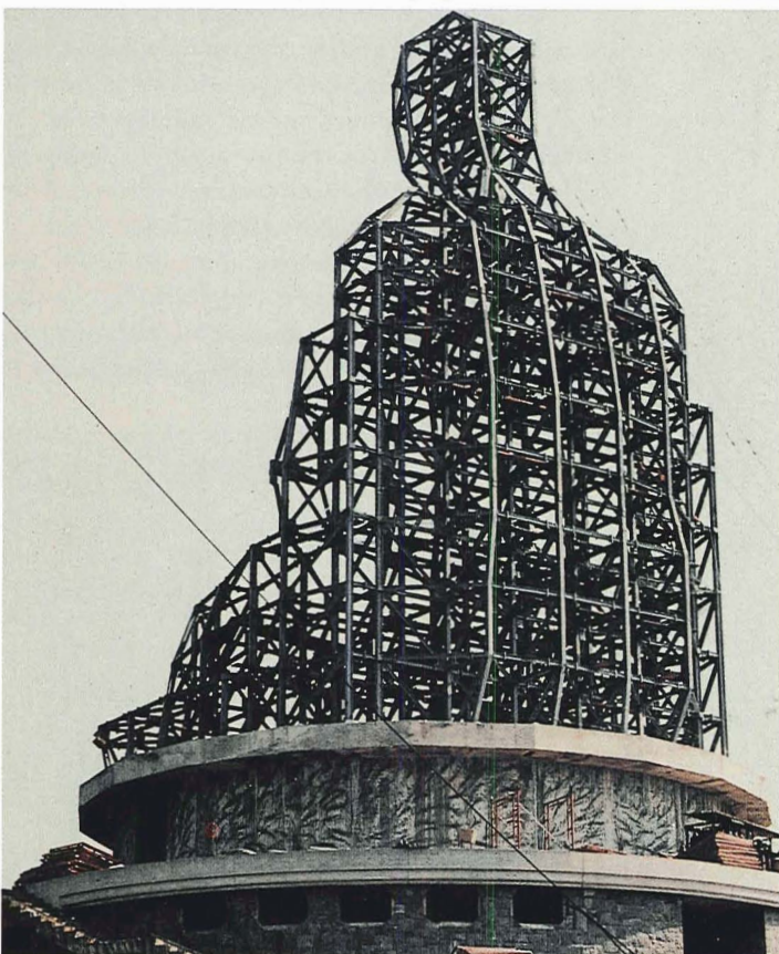
At top and in closeup above is Hong Kong's mammoth Po Lin Buddha, shown under construction. The interior structure was coated with a spinoff IC 531 product that provides superior protection against corrosion and offers cost and environmental bonuses.
