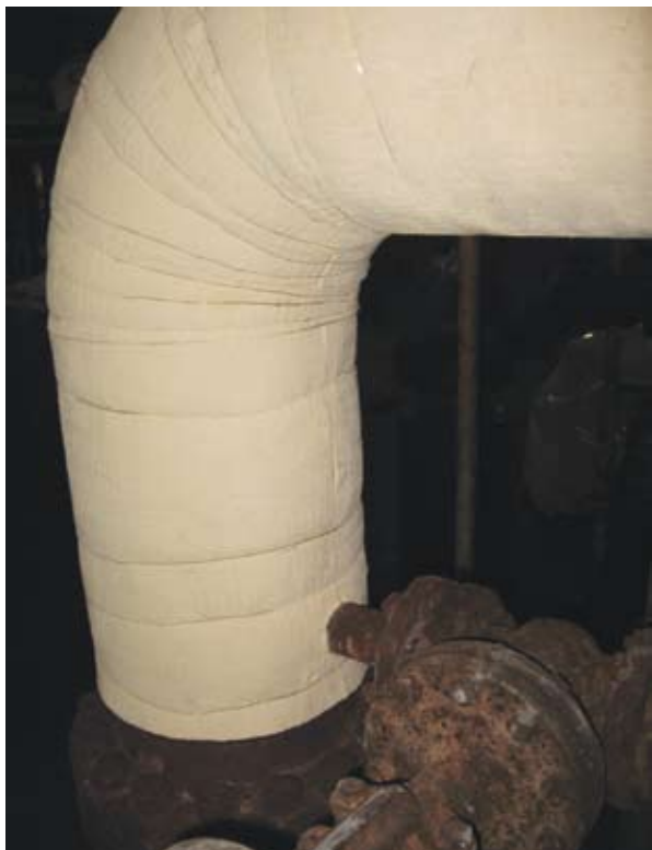
Flexible insulating blankets come in a variety of shapes and sizes, lending themselves to many different applications.
