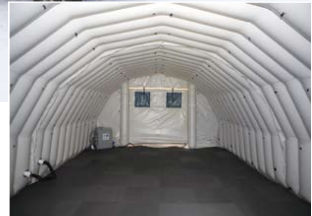
Resembling an inflatable Quonset hut, the habitat is insulated and heated, has power, and offers 384 square feet of living space.
