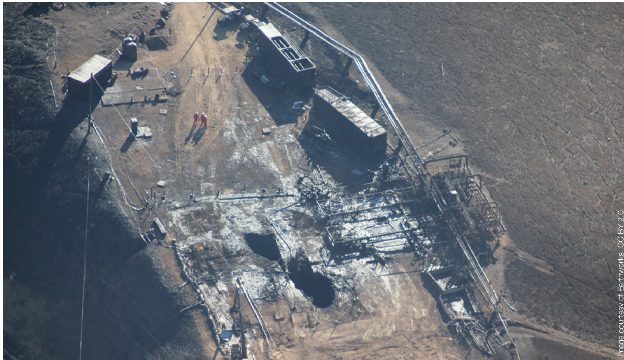
During a natural gas leak from this well in Aliso Canyon in late 2015 and early 2016, thousands of residents were relocated from the neighboring Los Angeles neighborhood of Porter Ranch. But thousands more were able to stay in place after Southern California Gas ordered 10,000 Air Scrubber Plus units and distributed them to residents. The devices are based on a more advanced form of an air purifier built for NASA in the 1990s, which breaks down organic contaminants in the air.
