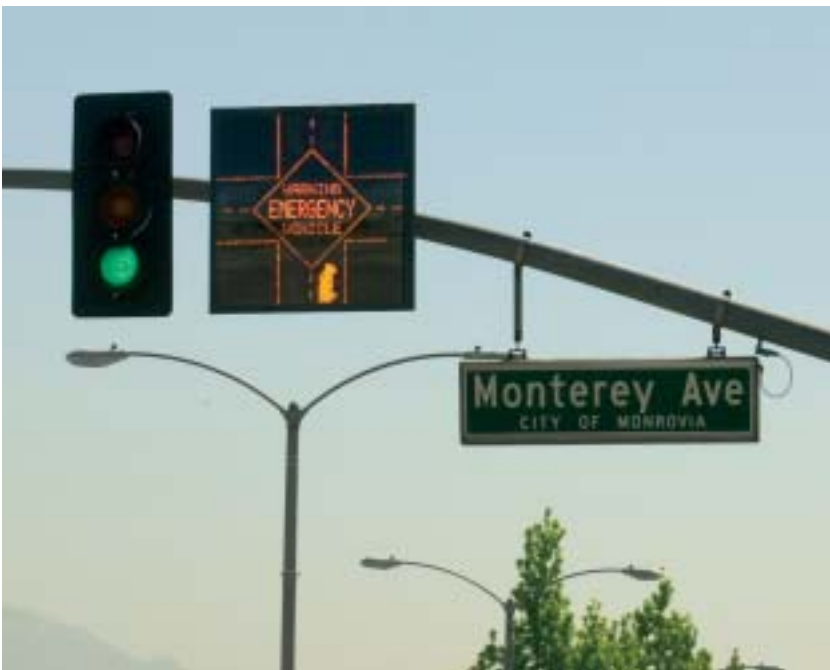
High-intensity light-emitting diode displays are positioned above the centers of intersections to inform motorists from which directions emergency vehicles are approaching.
