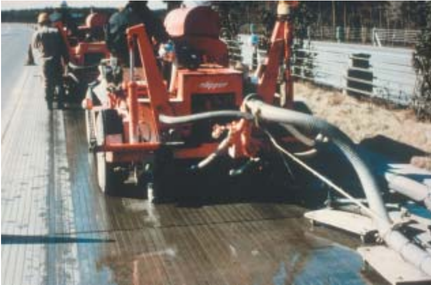
From the runway to the roadway, grooved surfaces in concrete significantly improve wet weather traction for stopping and steering.
