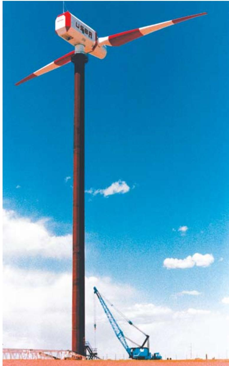
first multimewatt wind turbine, was developed—capable of providing electricity to thousands of homes. Successive experimental models (13 in all) were built throughout the country. Viterna notes that these were also record setting in size and output; the 4-MW capability of the WTS-4 turbine, built in 1982 in Medicine Bow, Wyoming, was not surpassed for about 25 years.
