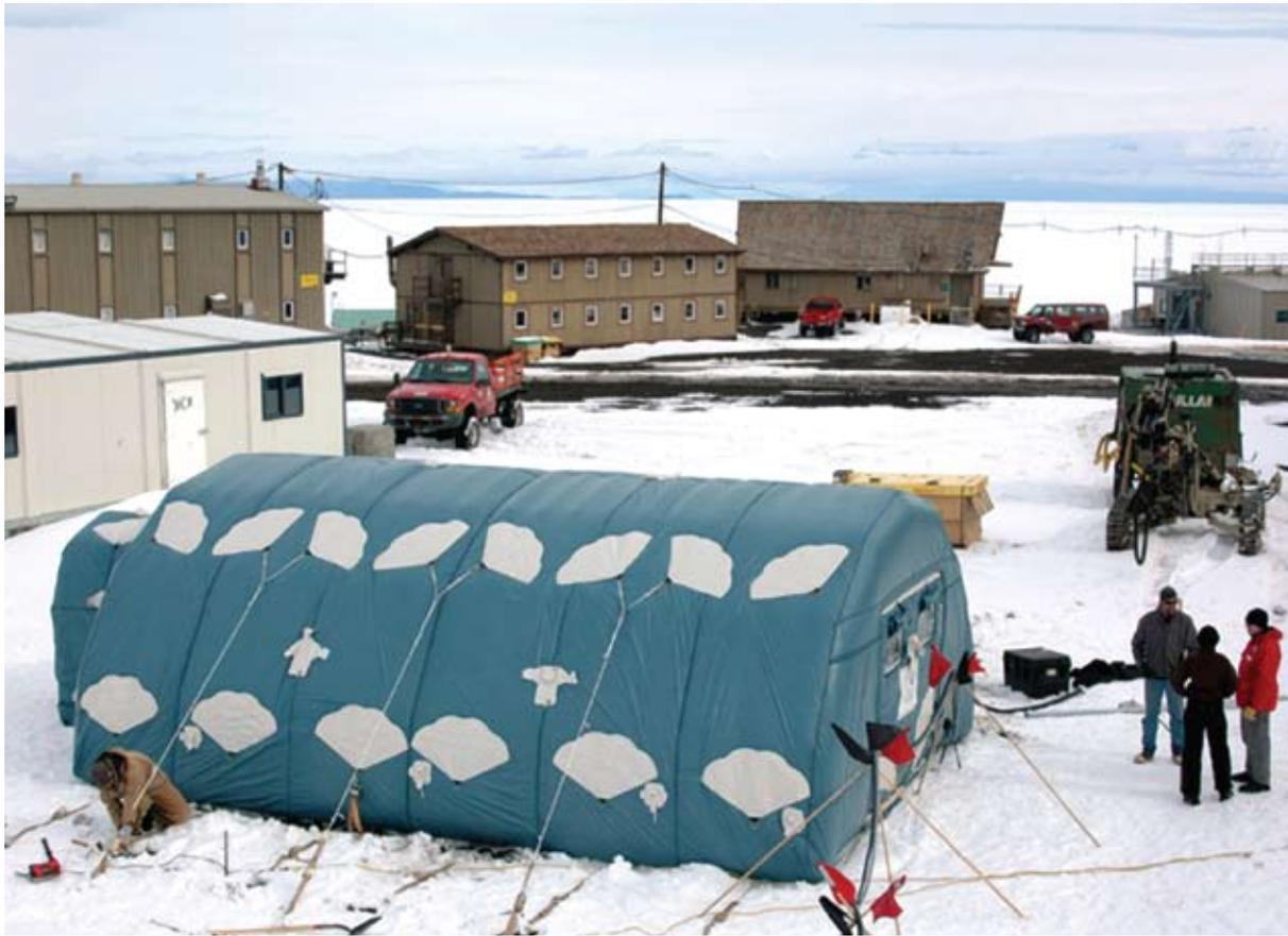
The prototype inflatable shelter tested at McMurdo Station in Antarctica demonstrated the promise of similar structures for use on the Moon. Such structures could also be ideal for mobile field hospitals in challenging environments on Earth.
