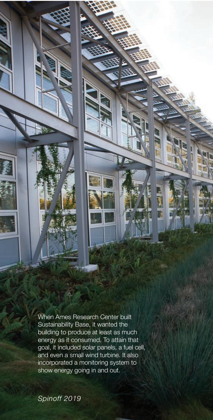
When Ames Research Center built Sustainability Base, it wanted the building to produce at least as much energy as it consumed. To attain that goal, it included solar panels, a fuel cell, and even a small wind turbine. It also incorporated a monitoring system to show energy going in and out.
