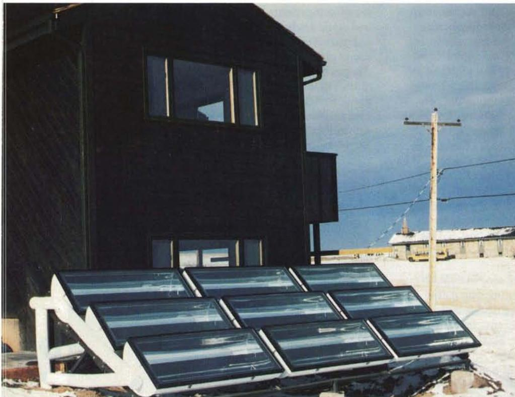
*A spinoff coating helps control "outgassing"—material burnoff—in solar collection systems, thereby preventing loss of heat-collecting*
