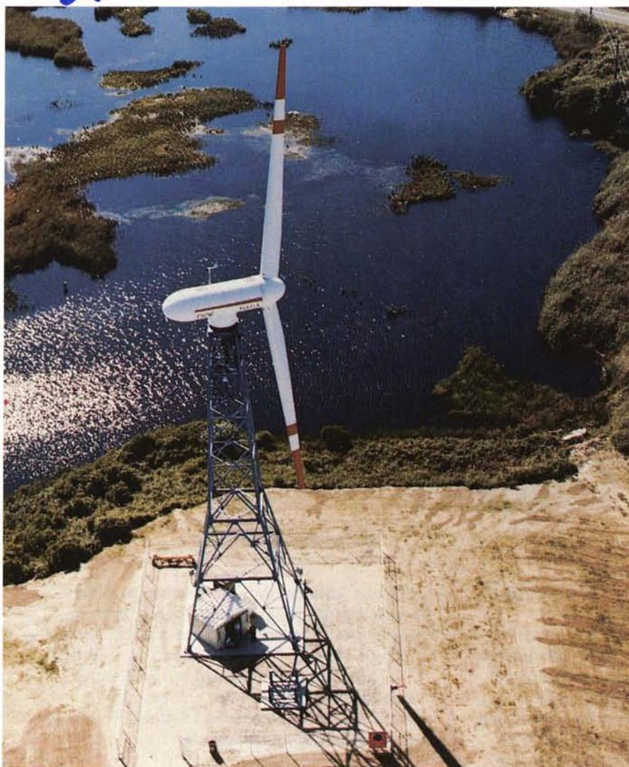
On a hill above the town of Boone, North Carolina, there is a structure resembling a gargantuan airplane propeller mounted atop a framework tower. A modern counterpart of the age-old windmill, it is a wind turbine generator which harnesses the power of the wind to produce two million watts of electricity, enough to serve the needs of several hundred homes.
