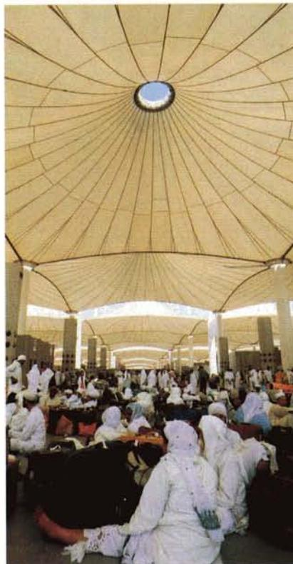
Although temperatures outside sometimes reach 130 degrees, it is a comfortable 80 under the "big top;" the coated fabric roof reflects 75 percent of the Sun's radiation and a unique open-sided, open-top tent design promotes cooling air circulation.
