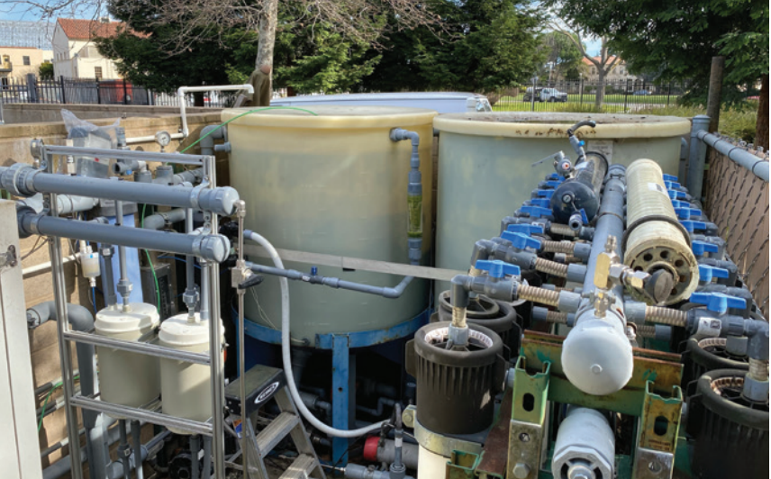
In the gray water reclamation system at Ames Research Center’s Sustainability Base, the two beige Aquaporin HFFO14 forward-osmosis modules on the left have as much filtration capacity as the entire legacy system on the right. Credit: Aquaporin A/S
